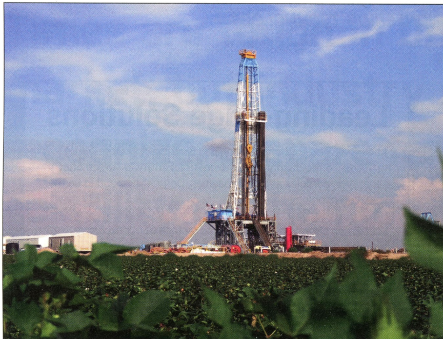
TOP: Latshaw Rig 8 drills in West Texas in September 2015. The 2,000-hp SCR rig is working for Element Petroleum in Howard County. Despite the industry perception that AC rigs are generally better performers than SCR rigs, Latshaw Drilling has found that there is still a place for SCR rigs. Latshaw Drilling has been able to put seven SCR rigs back to work since May 2015.
